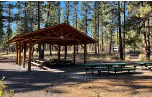
Picnic Shelter at Shevlin Park
