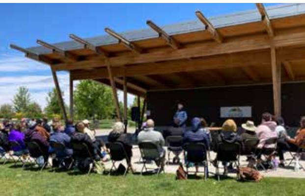
Picnic Shelter at Riverbend Park
