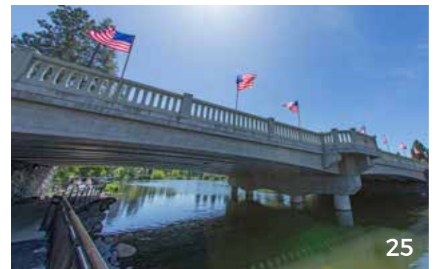
▼ Below photo: Newport Ave. bridge and undercrossing.
