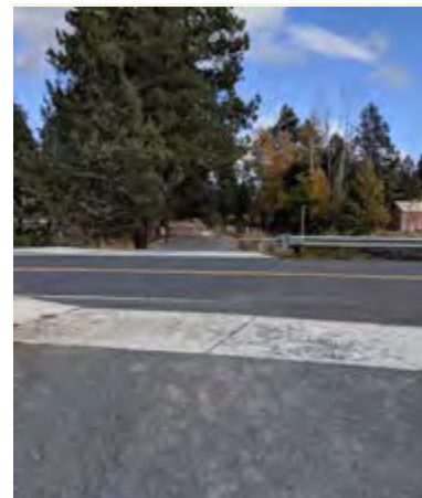
In an effort to improve the safety of the Central Oregon Historical Canal Trail, BPRD is using grant funds to add safety upgrades to Blakely Road, Brosterhous Road and Ferguson Road crossings.
